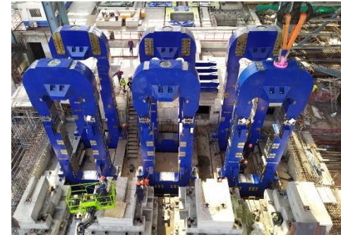
Dolvi Phase-III: Roughing Mill Housing erected
