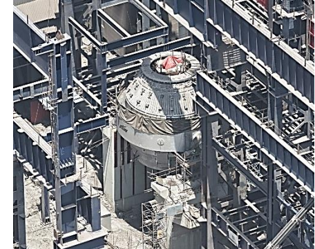
Dolvi Phase-III: BoF-3 Converter with top cone erection under progress
