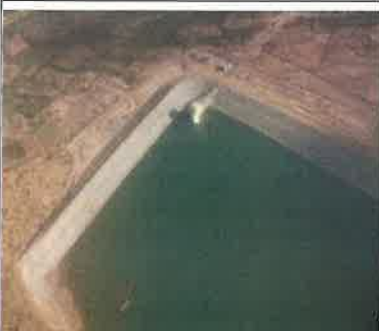
Raw water reservoir (35 Mn m3)
