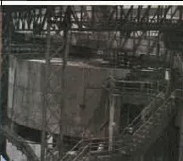
CO2 injection system at SMS
