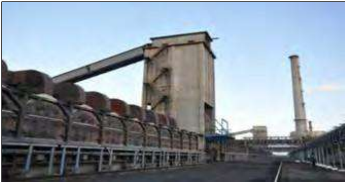
COKE OVEN PLANT
