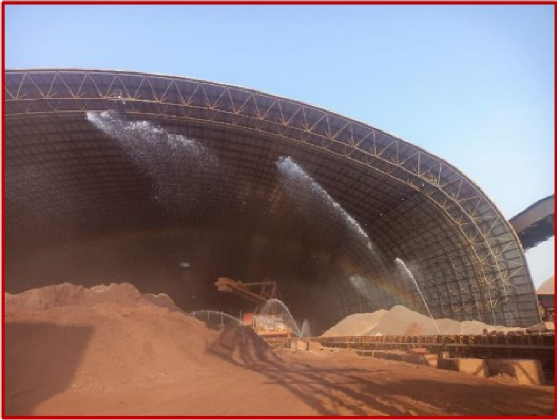
Location - Ore & Flux Yard
