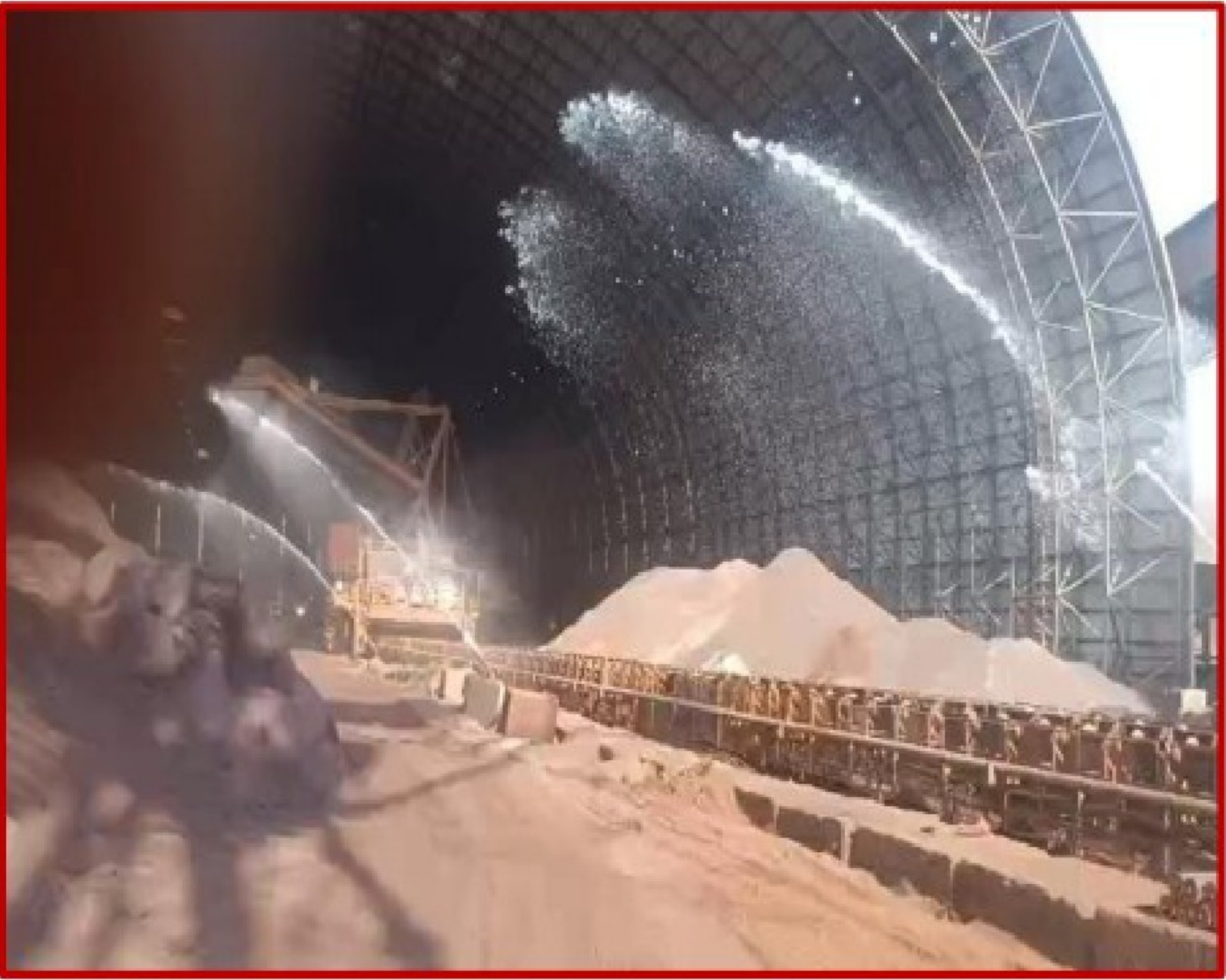
Location - Ore & Flux Yard
