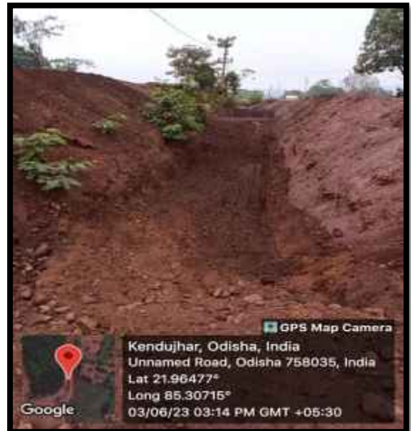
Series of settling pit
