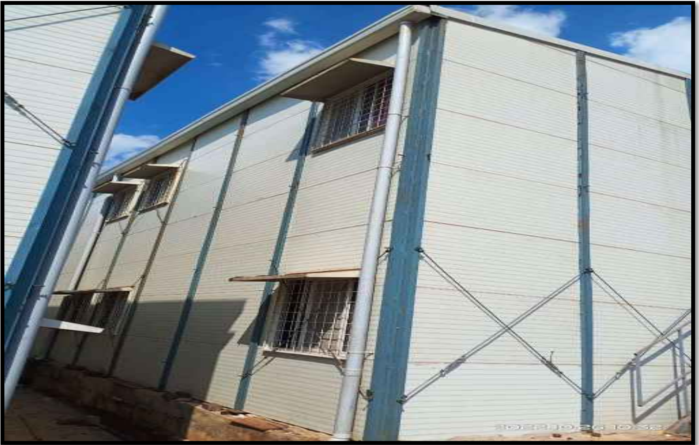
ROOFTOP RAINWATER HARVESTING AT OPERATOR'S COLONY
