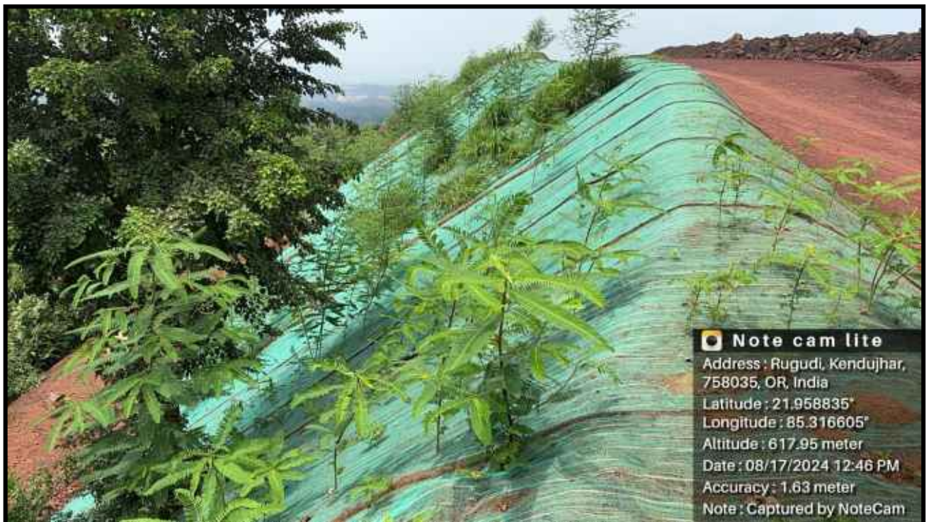
Coir matting at Katesahi OB dump area
