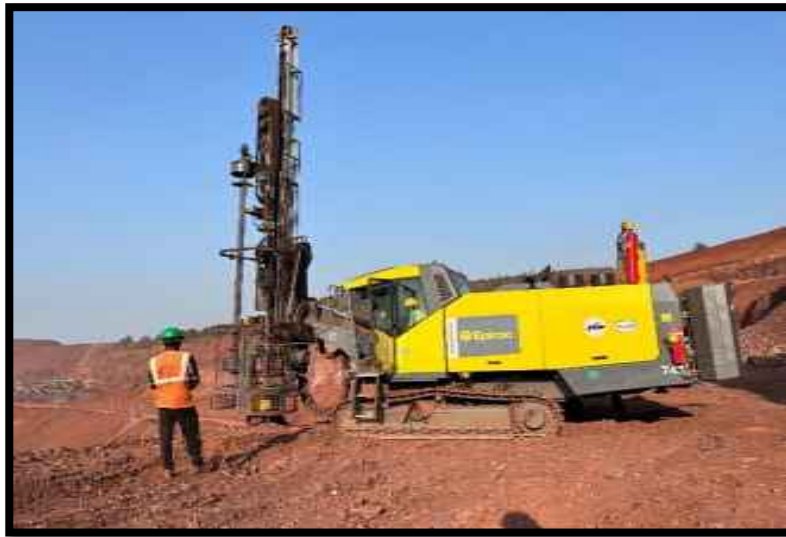
Wet Drilling and Dust Extractor System in Drilling Operation
