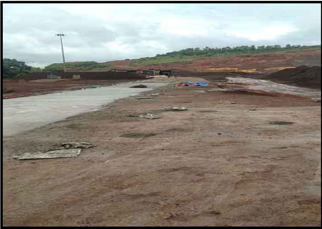
CC ROAD AT MDH AREA
