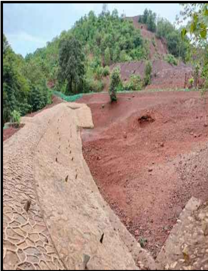
KANHUSAHI RAINWATER HARVESTING OF DIMENSION (50m*60m*2m)
