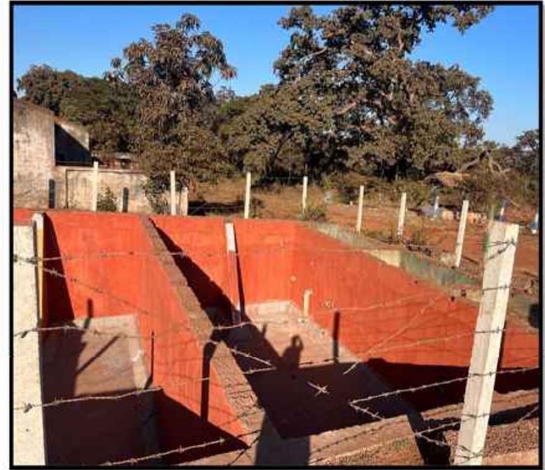
Collection pit of Rooftop Rain water harvesting
