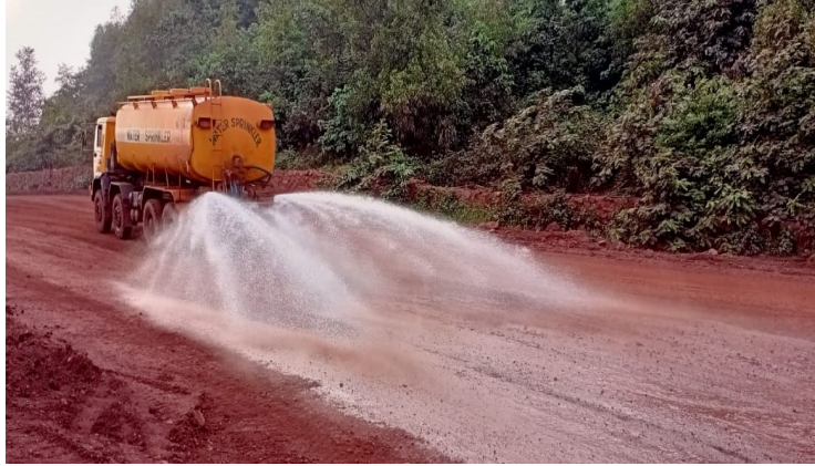
Water Tanker Arrangement for Haul Road Dust Suppression
