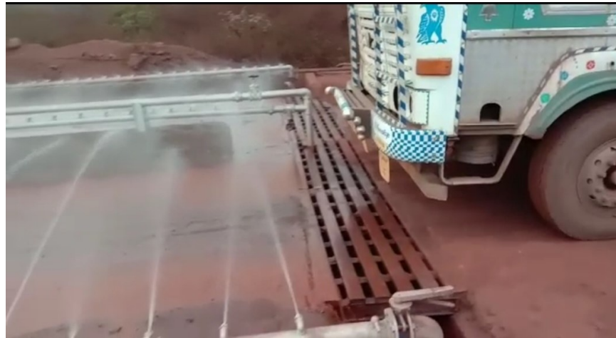
Wheel Washing System near Gate No 6.
