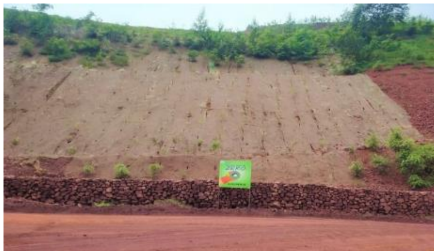
Retaining Wall, GeoCoir Matting & Plantation on Backfilled Area 2
