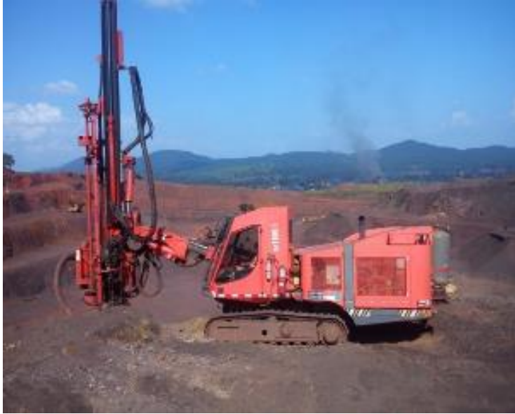
Wet Drilling and Dust Extractor System in Drilling Operation
