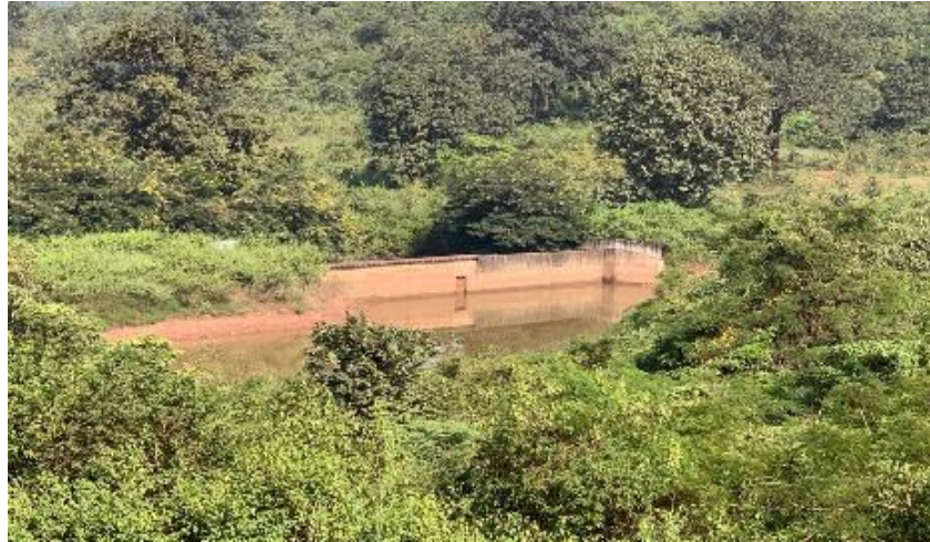
Check Dam near railway siding
