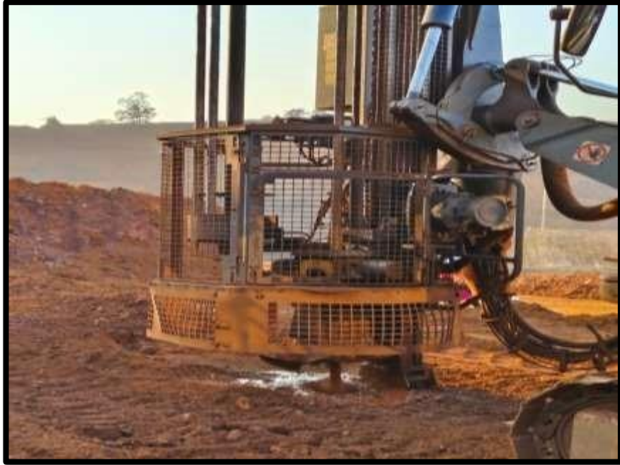
Wet Drilling System in Drilling Operation
