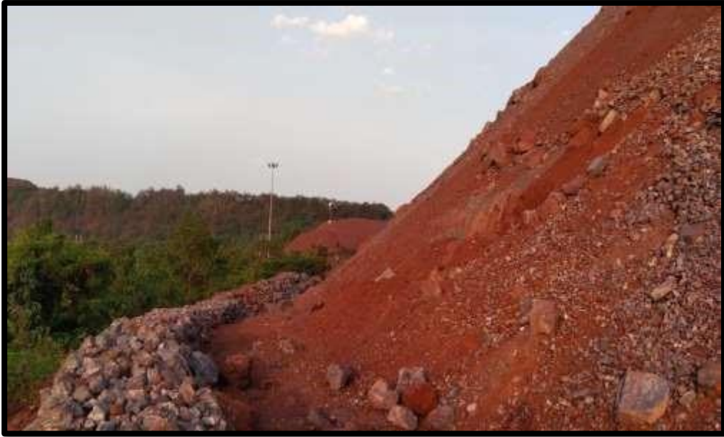
Retaining Wall
