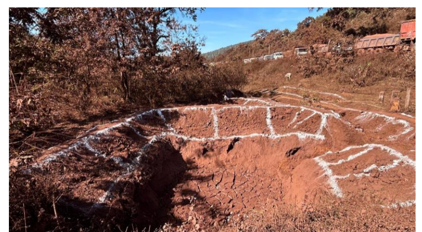
Check Dams & Settling Pond
