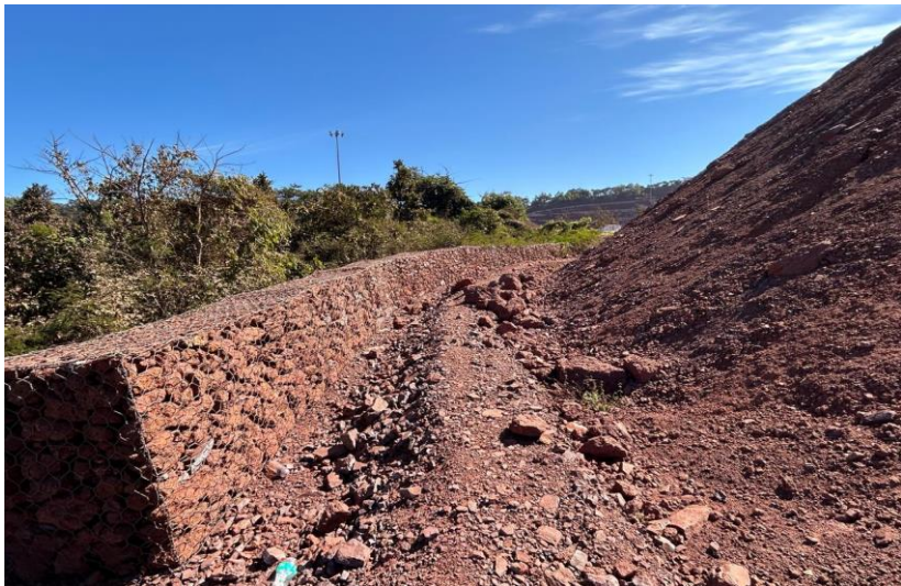
Retaining Wall
