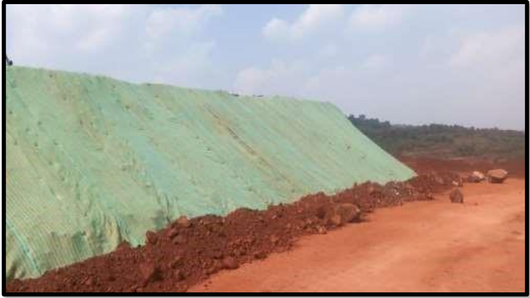
Coir Matting on Dump
