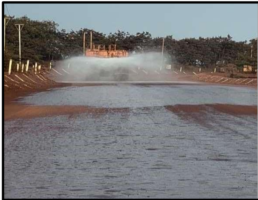
Water Tanker Arrangement for Haul Road Dust Suppression
