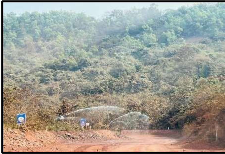
Fixed water sprinkling arrangements
