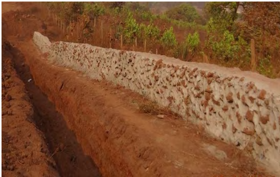
Retaining wall/ Garland drain
