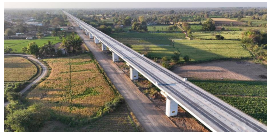
MAHSR Viaduct at Anand District, Gujarat
