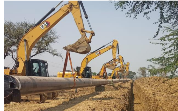
Slurry Pipeline laying in Odisha
