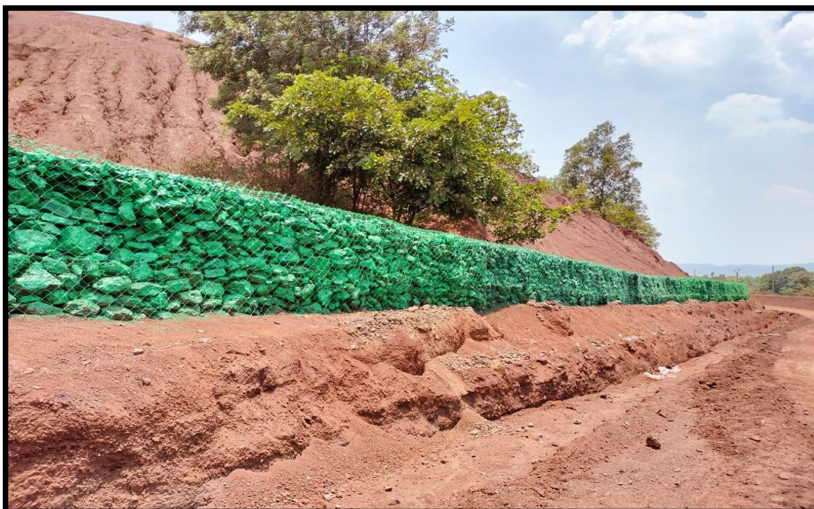
Retaining Wall at MDH
