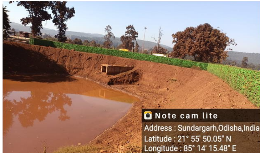
Settling Pond near Gate 2
