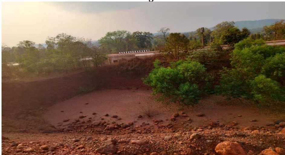
Settling Pond near Quarry 5
