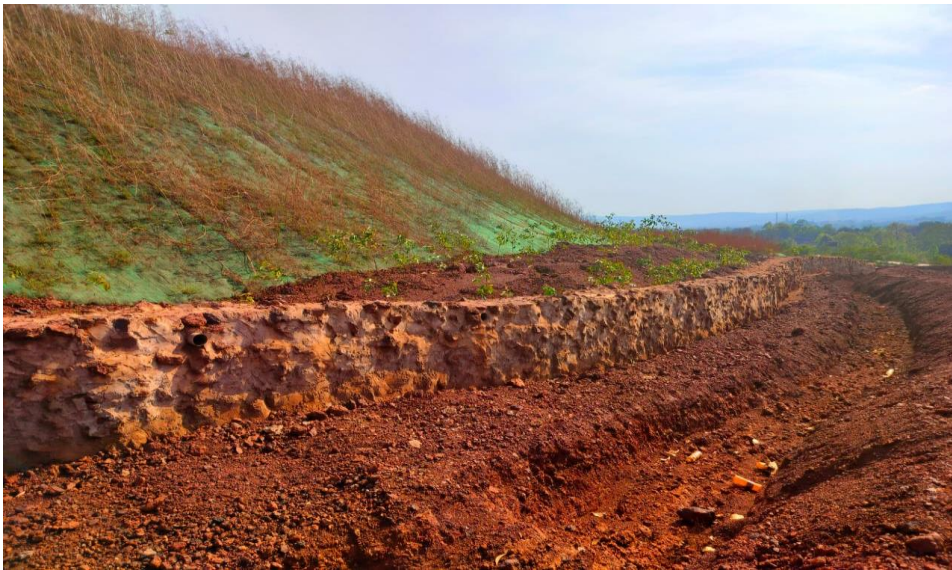
Retaining Wall
