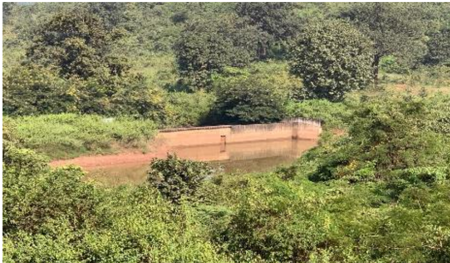
Check Dam near railway siding
