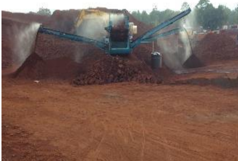
Dry Fog System in Mineral Handling Plants
