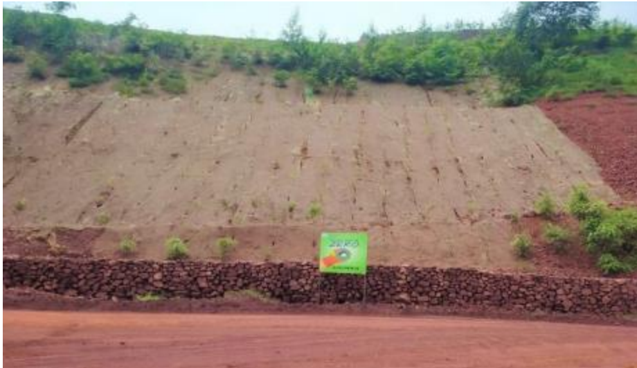
Retaining Wall, Coir Matting & Plantation on Backfilled Area 2
