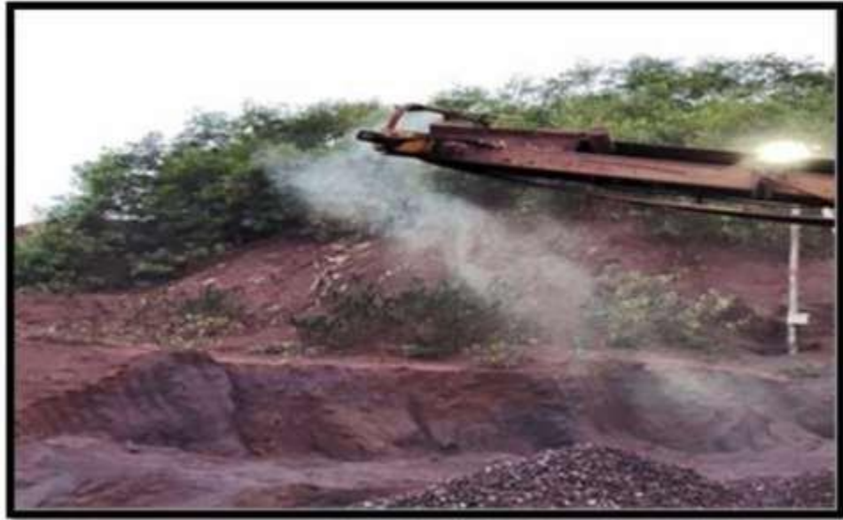
Dry Fog System in Mineral Handling Plants
