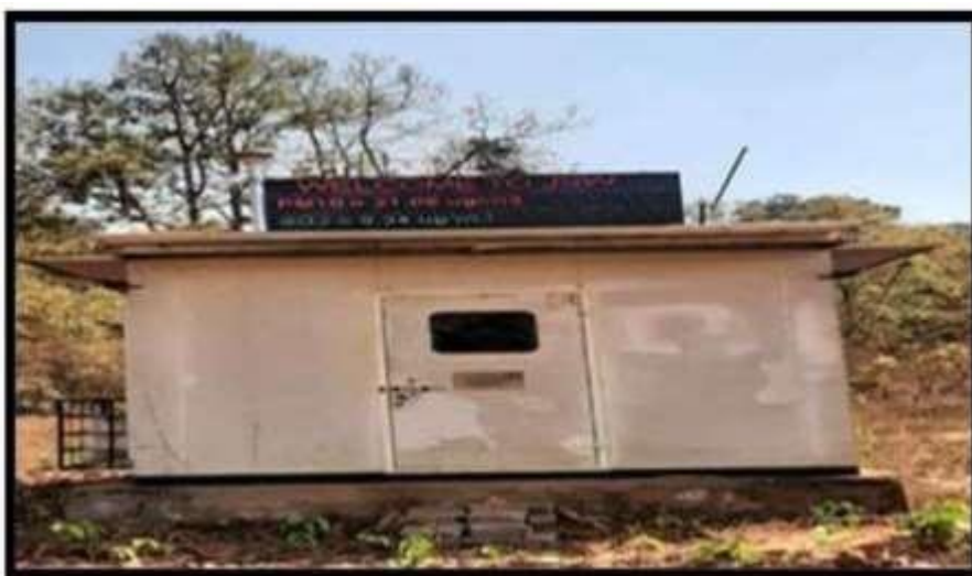
CAAQMS Near Pump House
