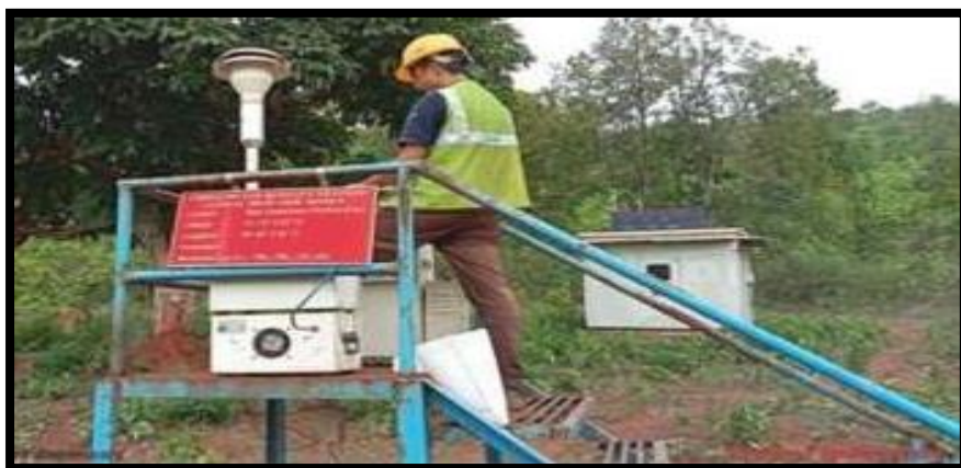
AAQ Station Near Pump House
