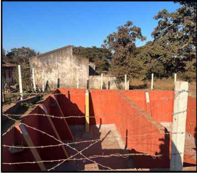
Collection pit of Rooftop Rain water harvesting
