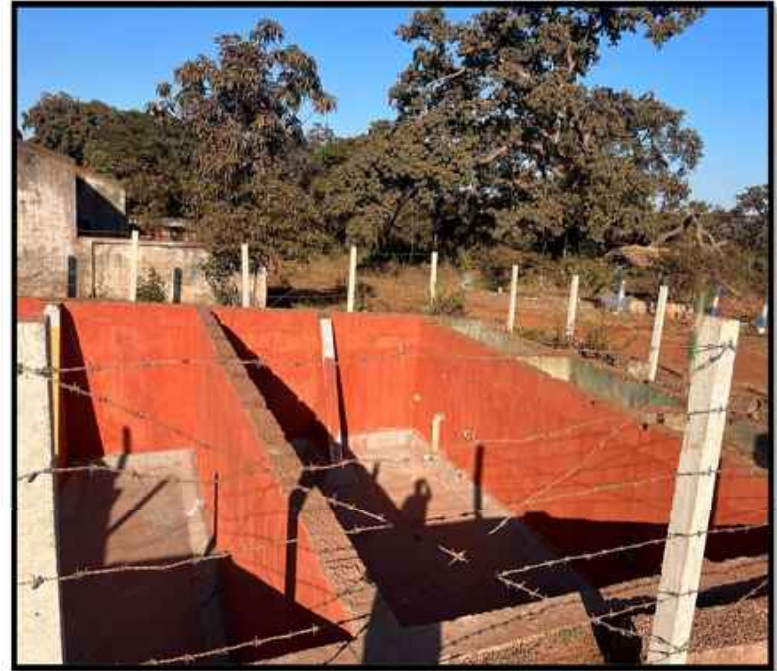
Collection pit of Rooftop Rain water harvesting
